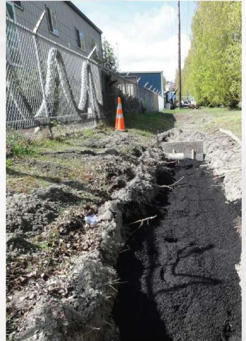
*Figure 2: The Port of Port Townsend is using biochar to filter heavy metals in a below-grade swale. The galvanized fence in this photo is one of the boatyard's primary sources of zinc. (Image courtesy Francesco Tortorici)*
