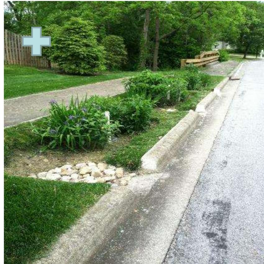
Bioretention facility overwhelmed by sediment,
