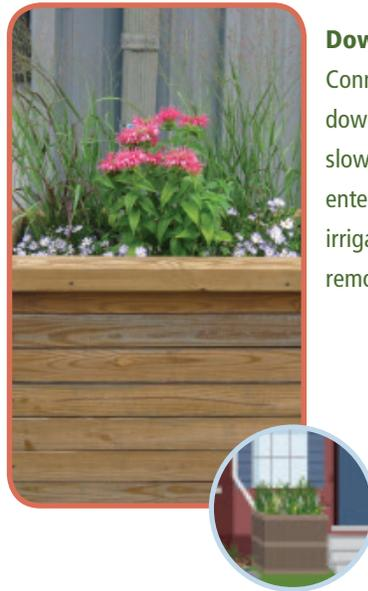
**Downspout Planter:** Connected to the roof downspout, these planters slow water down before entering the sewer while irrigating plants and removing pollutants.
