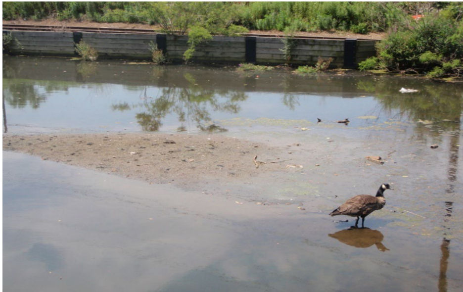
Sediment accretion in the Manayunk Canal at Leverington Street and Domino Lane (2011)
