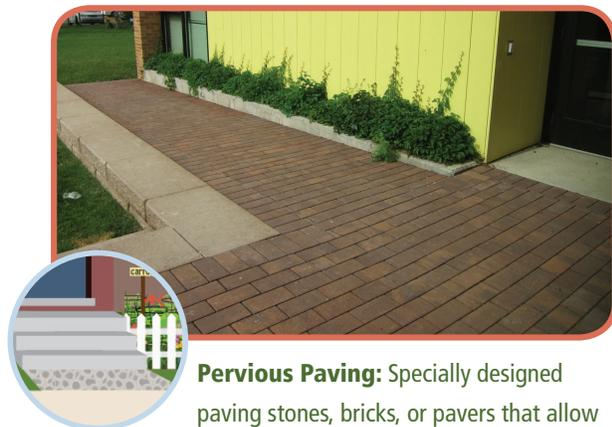
**Pervious Paving:** Specially designed paving stones, bricks, or pavers that allow water to soak into the ground below.
