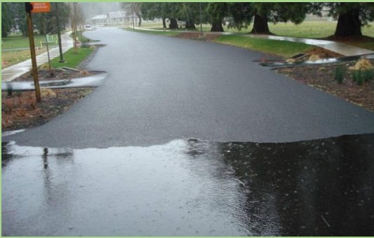
Porous Asphalt (top) vs. traditional asphalt (bottom) (Source: vaasphalt.org )
