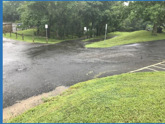
(Left) Runoff from the front entranceway flows towards the creek via the driveway and adjacent swale. (Right) Evidence of erosion was observed on the backside of the school.
