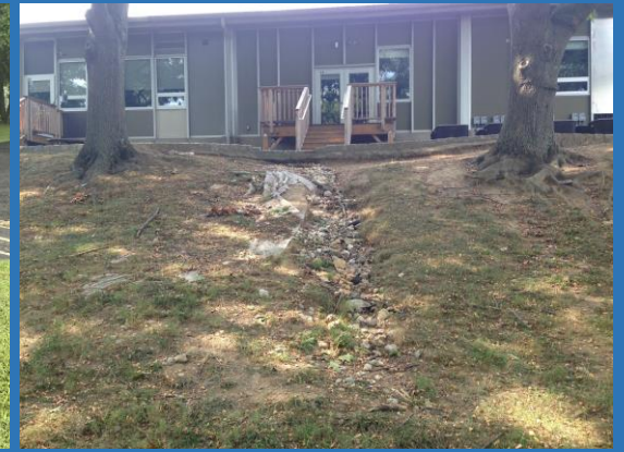
(Left) Runoff from the front entranceway flows towards the creek via the driveway and adjacent swale. (Right) Evidence of erosion was observed on the backside of the school.
