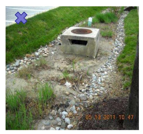
Bioretention facility overwhelmed by sediment, Stormwater Maintenance, LLC, 2011
