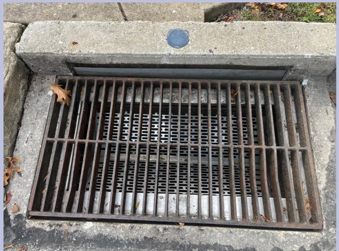
Workshop participants viewed 2 adjacent stormwater inlet filters in Upper Merion Township's parking lot. The **top** was awaiting maintenance whereas the **bottom** had recently undergone routine seasonal maintenance. The comparison highlighted the importance of maintaining these structures in the fall months, to minimize pipe clogging and sedimentation.
