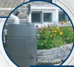
A rain barrel collects stormwater.
